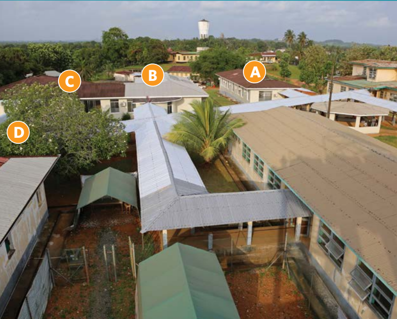
PIH made major infrastructure changes to J.J. Dossen Hospital. Photo by Rebecca E. Rollins
