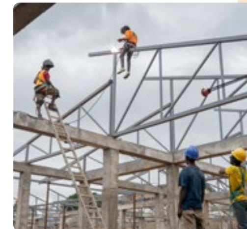
Construction of the North Ward of the MCOE. Photo by Chiara Herold / PIH
