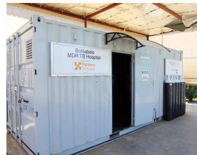
The pressure swing adsorption oxygen plant at Botsabelo MDR-TB Hospital, Maseru, Lesotho Tom Patterson/PIH
