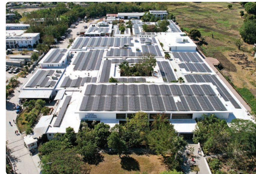
An aerial view of the solar panel system on the roof of Hôpital Universitaire de Mirebalais. Photo by Thierry Prinston / PIH
